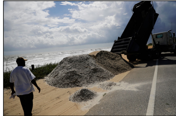
b) Placing fill material to protect a roadway in Flagler County from damage 26 .
