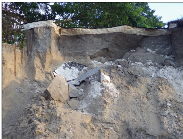
Figure 44. Washout at the West Orange Trail Surface (Latitude 28°41'8.70"N / Longitude 81°30'20.79"W).
