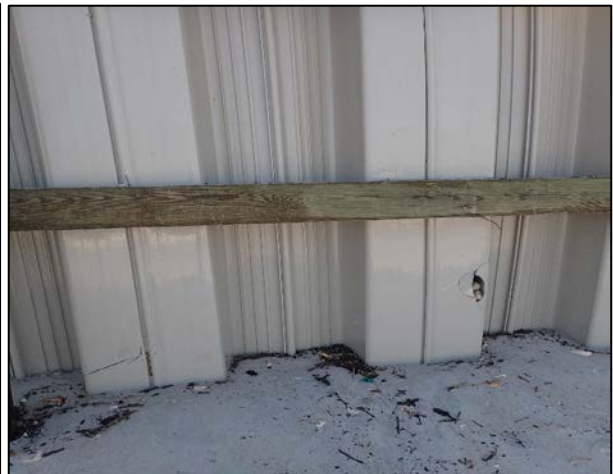
b) Cracking and hole in sheet pile material (Latitude 29°56'44.79"N / Longitude 81°18'7.05"W).
