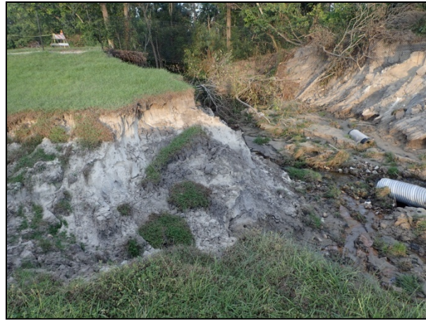
Figure 48. Erosion lateral to the main channel likely from failed drainage structure 3 (Latitude 28°41'9.15"N / Longitude 81°30'21.64"W).
