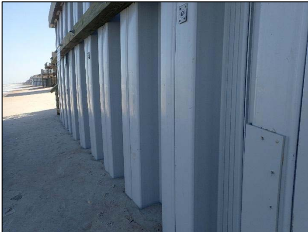
a) Wall bowing below wale and anchors (Latitude 29°57'46'1.08"N / Longitude 81°18'12.22"W).
