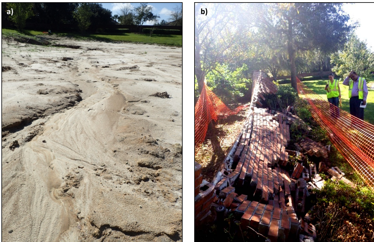
Figure 16: a) Erosion from overland flow within the retention area, where the direction of water flow was from sinkhole "A" toward sinkhole "B" (Latitude 29°40'48.47"N / Longitude 82°29'43.94"W), and b) toppled brick wall over a 12.5 m length at sinkhole "E" (Latitude 29°40'25.12"N / Longitude 82°29'48.35"W).
