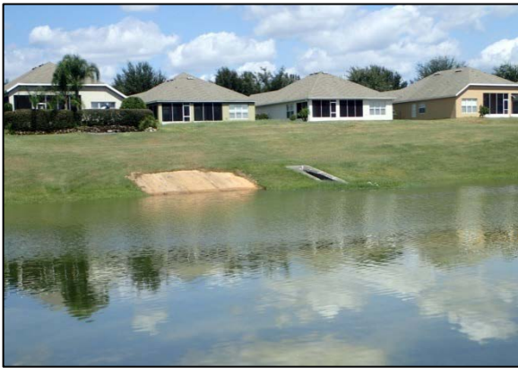
Repaired sinkhole A
