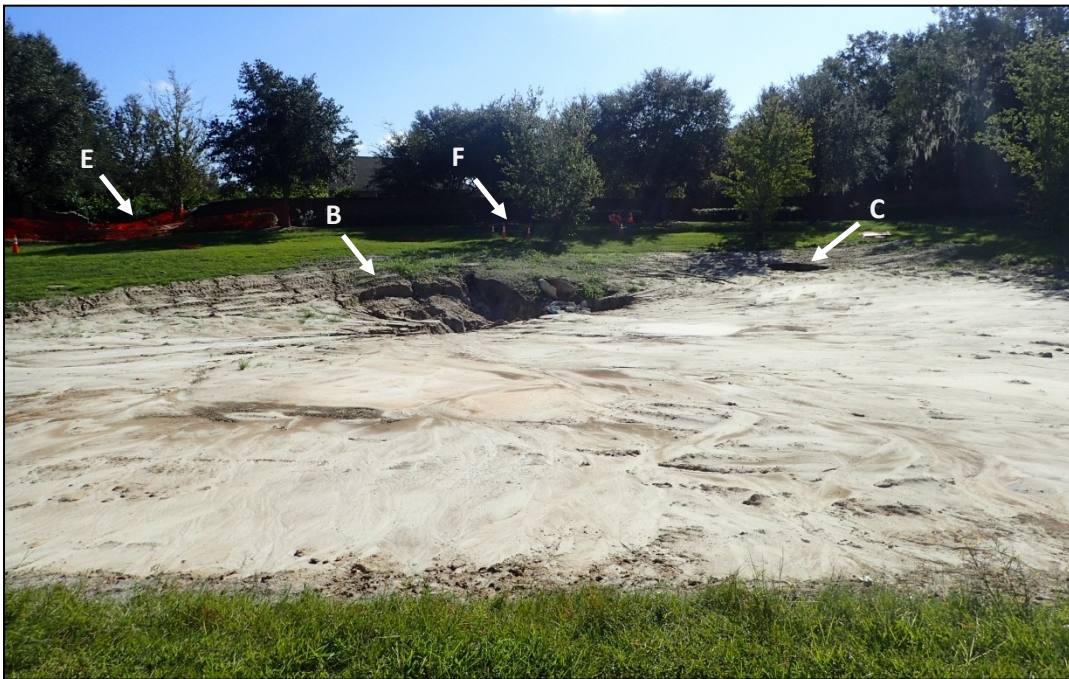
Figure 11: Image of the retention pond showing the locations of sinkhole "B" with the drainage outfall, sinkhole "C", sinkhole "E" under the brick wall of the community, depression "F", and evidence of the of water flow into sinkhole "B" in the retention pond foreground from the storm event (Latitude: 29°40'48.05"N / Longitude: 82°29'43.61"W).
