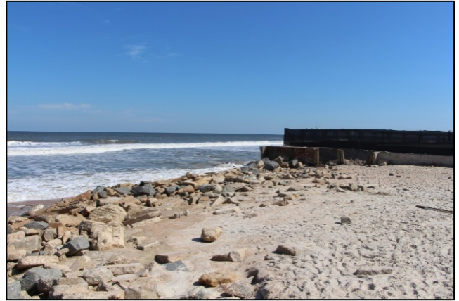
d) Overwash and unravelling of poorly constructed revetment (approximate location Latitude 29°51'34.61"N / Longitude 81°15'57.22"W).
