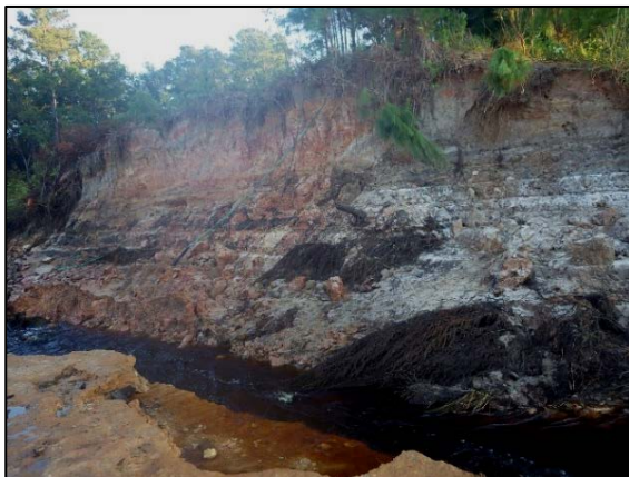
c) Scour of the east embankment of the dam (Latitude 30°46'33.89"N / Longitude 81°58'15.47"W).
