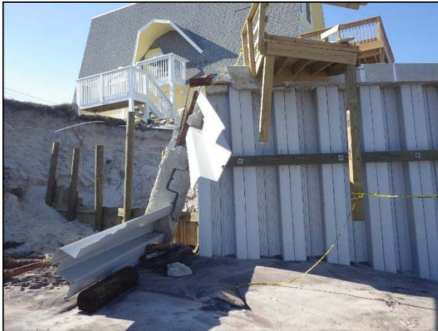
a) South wing wall destroyed.
