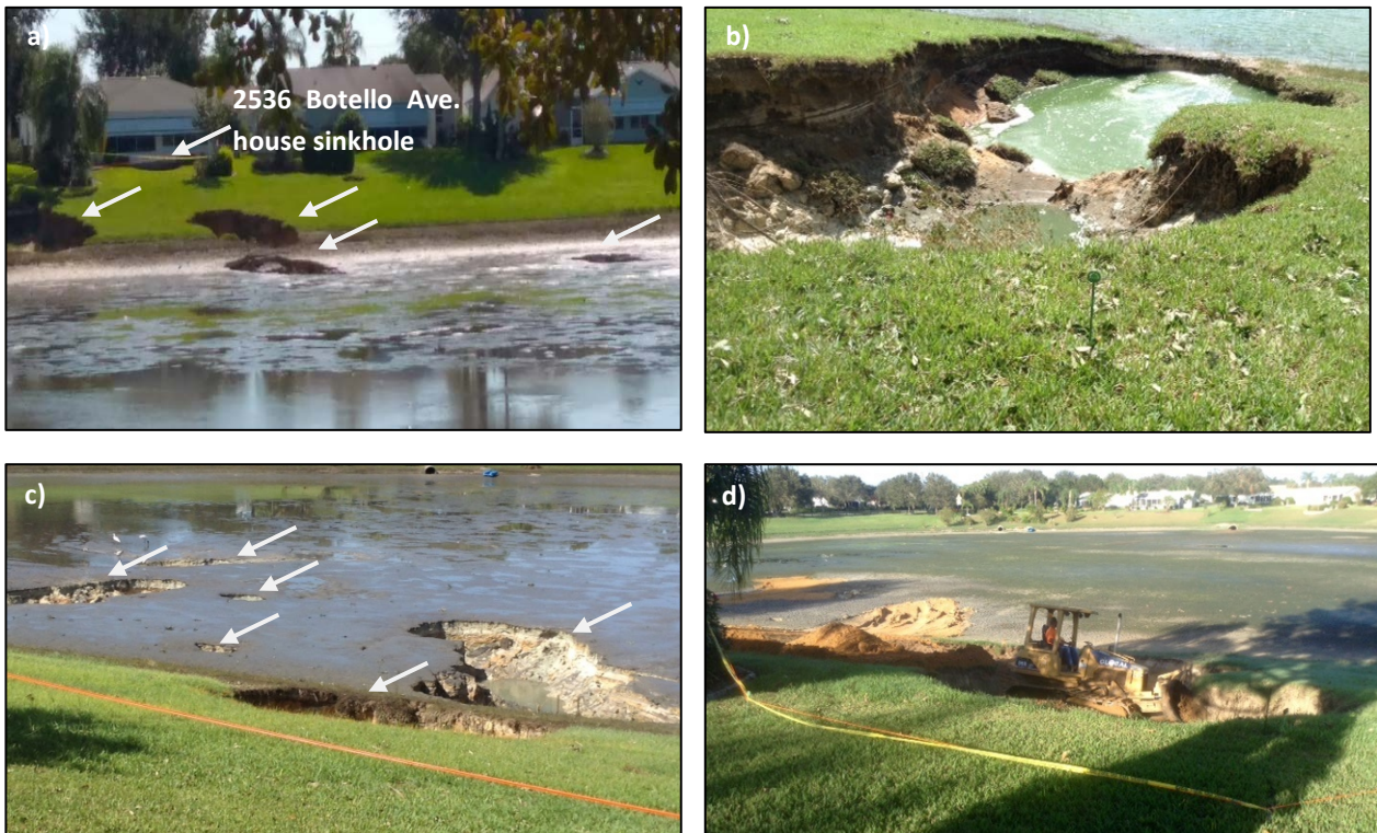
Figure 36. Sinkholes on the bank of, and within the retention pond between Alhambra Way and Botello Ave. (a, b, c), and under repair (d) (Latitude 28°57'11.92"N / Longitude 81°59'31.49"W) (images courtesy of local residents Sheila Huffman Dailey, Dan Snyder, and Barbara Beveridge).
