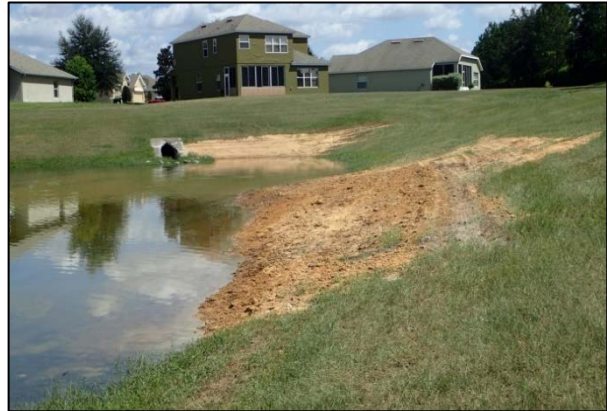
Repaired sinkhole B (back) and C (front)
