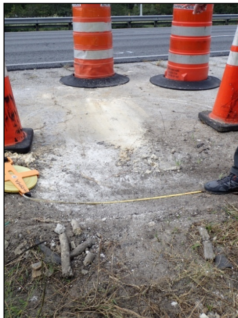
Figure 20: Distress from a repaired sinkhole approximately 1 m diameter at the roadway edge of the northbound lane of I-75 (Latitude 29°39'7.99"N / Longitude 82°24'44.00"W)
