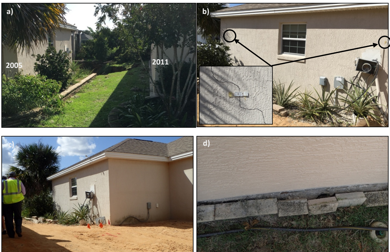
Figure 30: Documentation of a sinkhole that formed between homes at 2005 and 2011 Markridge Loop, The Villages, FL., including: a) the open sinkhole (dimensions unknown; pers. comm. Doug Wernicke); and b) cracks on the wall of 2005 Markridge Loop with crack gages; c) area between the two homes; and d) evidence of ground subsidence and an irrigation system at the wall of 2011 Markridge Loop after sinkhole backfilling. (Latitude 28°53'0.57"N / Longitude 82° 0'1.02"W).
