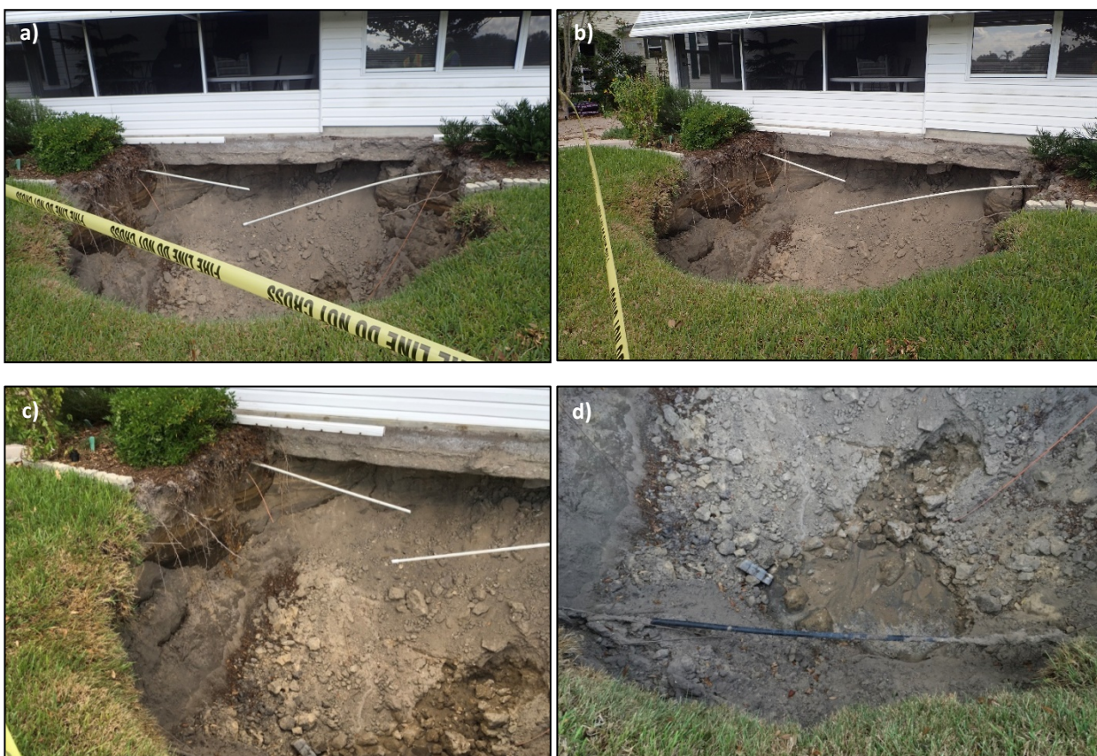
Figure 38. Sinkhole undercutting a foundation at 2536 Botello Rd. showing multiple front views (a, b, c,) and bottom of the sinkhole (d). (Latitude 28°57'11.67"N / Longitude 81°59'30.05"W).
