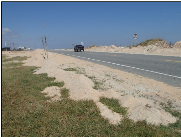
b) Windrows of washover deposits on west side of Highway A1A (Latitude 29°32'29.00"N / Longitude 81°9'25.0"W).
