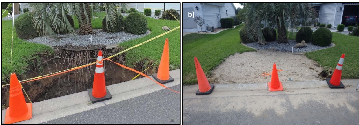
Figure 37. Sinkhole formed at 2532 Botello Avenue a) prior to repair 19 and b) following repair (Latitude 28°57'10.60"N / Longitude 81°59'30.50"W).
