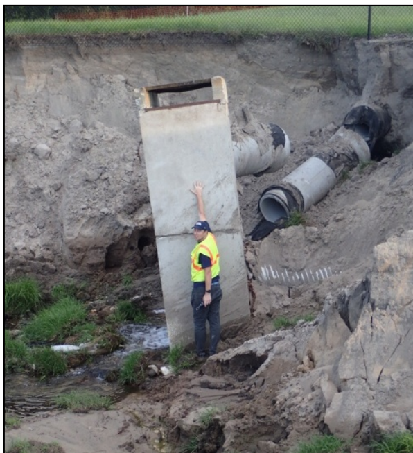
Figure 46. Damaged drainage structure 3, dimensioned by the investigators 2.4 m reach (Latitude 28°41'9.08"N / Longitude 81°30'22.39"W).
