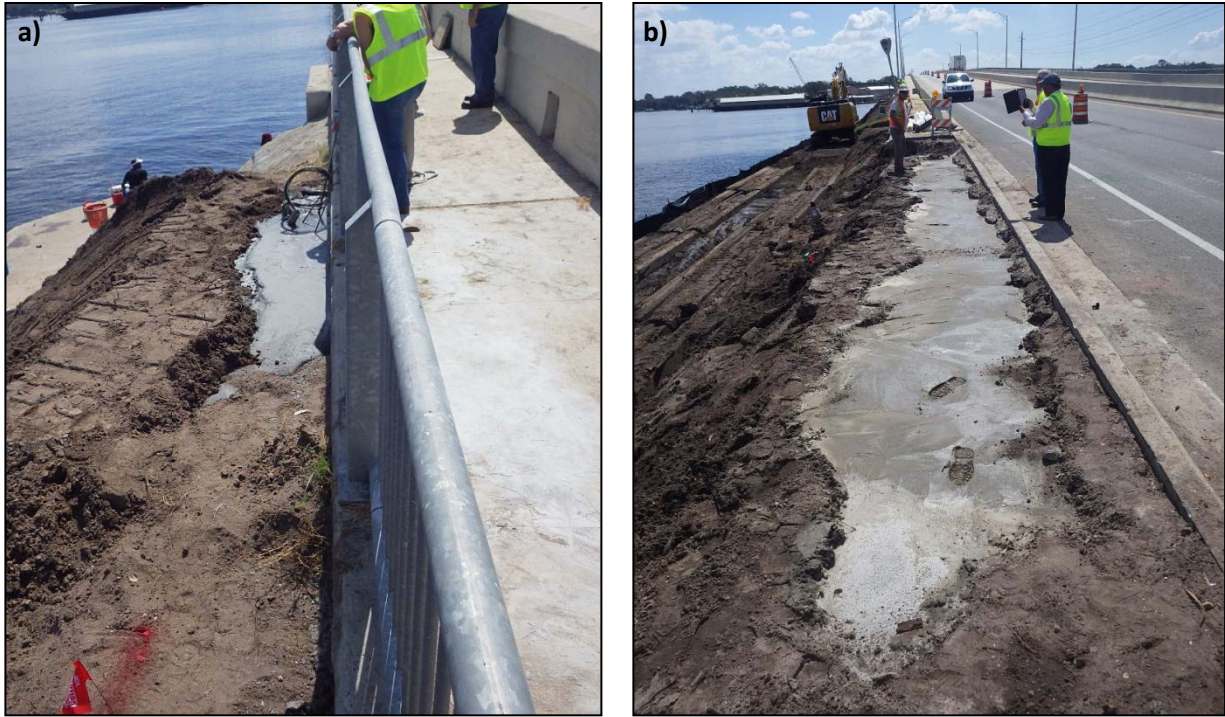
Figure 96. Repair of major scour damage along the northeastern bridge embankment of the US 17 bridge over the Trout River, (Latitude 30°23'45.44"N / Longitude 81°38'53.95"W) where the embankment was rebuilt and excavateable flowable fill trenches installed within the soil adjacent to the roadway to stabilize the roadway shoulder and underground utilities and protect against future erosion adjacent to the concrete covered stacked concrete sack wall near the northeast abutment (a) and along the eastern roadway edge to the north (b).
