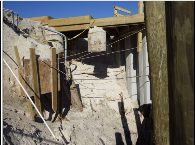
b) Damage behind the retaining structure.
