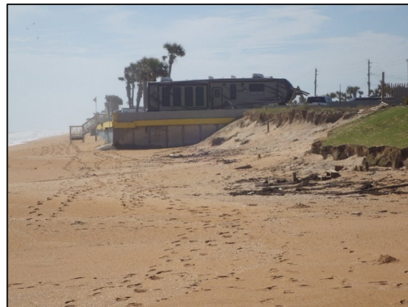
d) Scour on the north wing wall of the concrete seawall (Latitude 29°32'36.21"N / Longitude 81°9'30.17"W).
