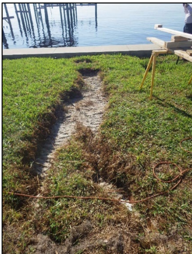
a) Localized scour behind the river bulkhead.
